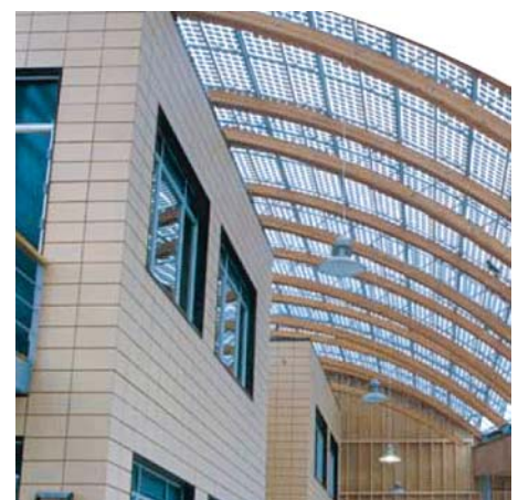
Figure 3. PV can be incorporated into glazing to provide shading and electricity.
