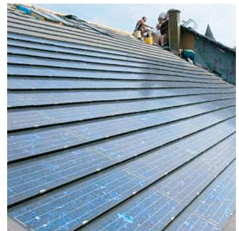
Figure 2. A PV roofing system
